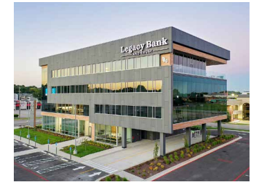
Legacy Bank and Trust Headquarters - Springfield, MO
