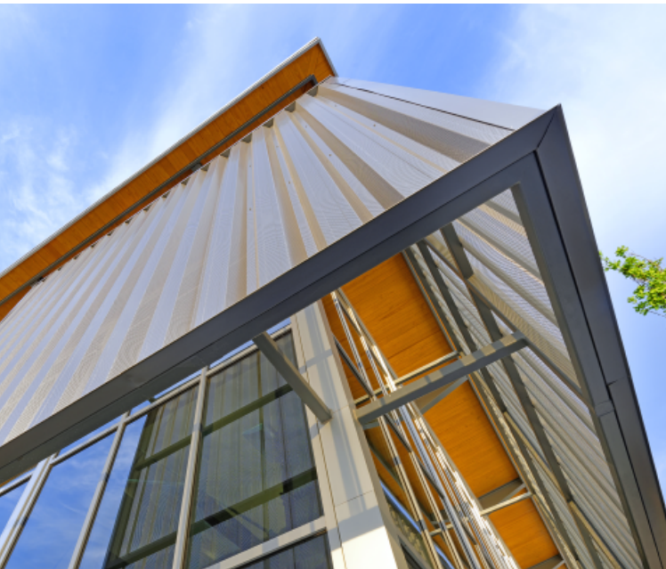
City Utilities Transit Center – Springfield, MO
